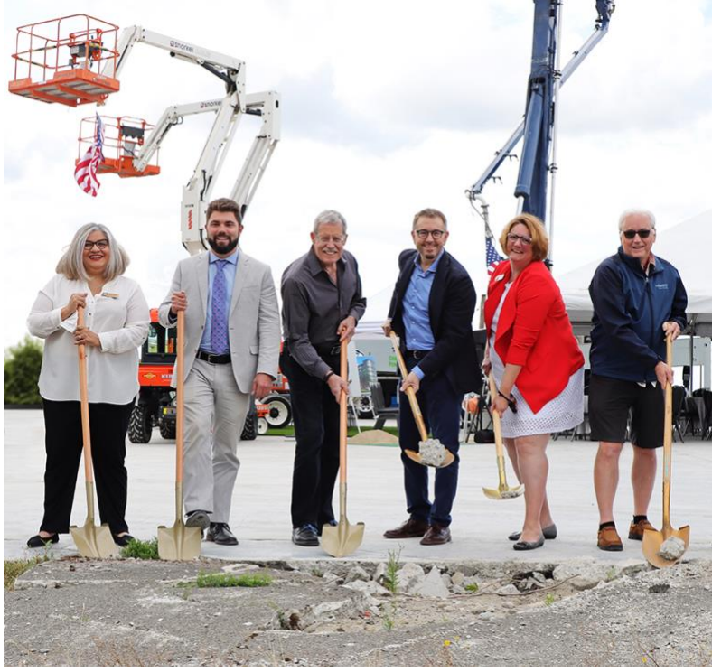
Helping kickoff construction of The Solera Project are (left to right) Councilmember Ruth Pérez, David Ratliff, president of DevCo LLC, Jack Hunden, founder of DevCo LLC, Mayor Armondo Pavone, Councilmember Angelina Benedetti, and Charles Seil, Planning Commission Vice-Chair.
